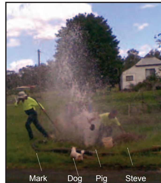
Pigging (cleaning) the water mains at Woomargama - April 2010 Mark McIntyre, Steve McIntyre, "Pig" & an excited dog...in action (Photo taken by Rory Winter on a mobile phone)
