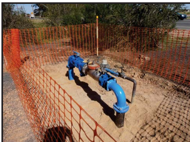
Installation of large fire service, Wagga Wagga
