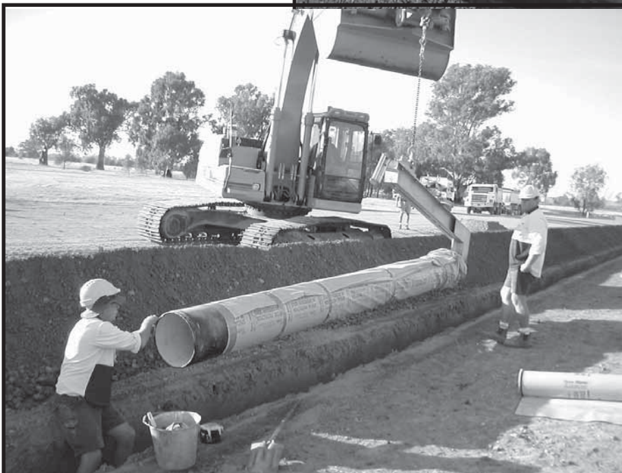
Construction of Bomen Rising Main Using 450mm sleeved ductile iron pipe
