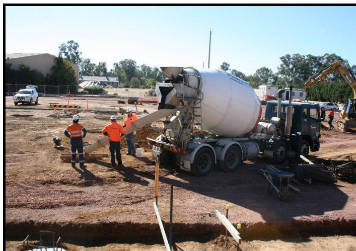
Pouring footings above and progress as at July 2015
