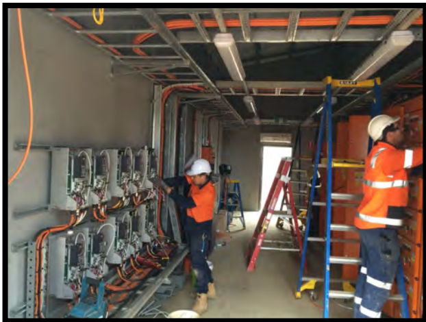
September 2016—Centrifuge Switchboard wiring
