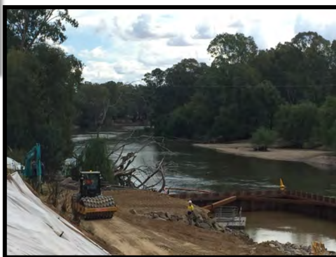
April—2017 Raw Water Intake Crane Pad construction
