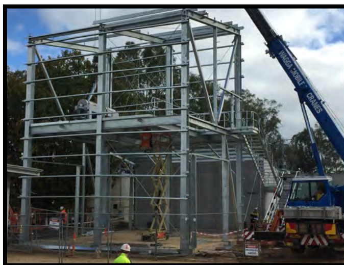
July 2016—Centrifuge being placed into position
