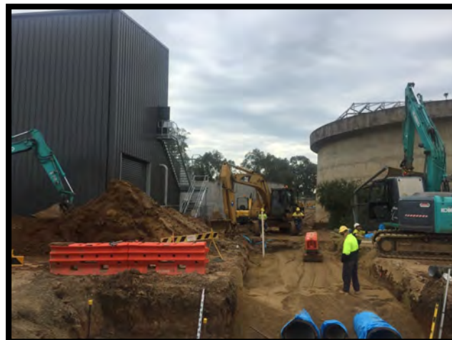
September 2016—Clearwater discharge piping crossing road
