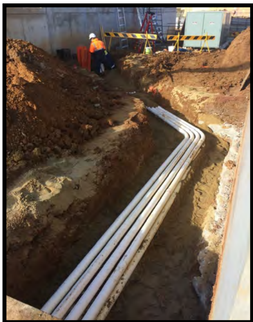
August 2016—Conduit installation adjacent to chemical building
