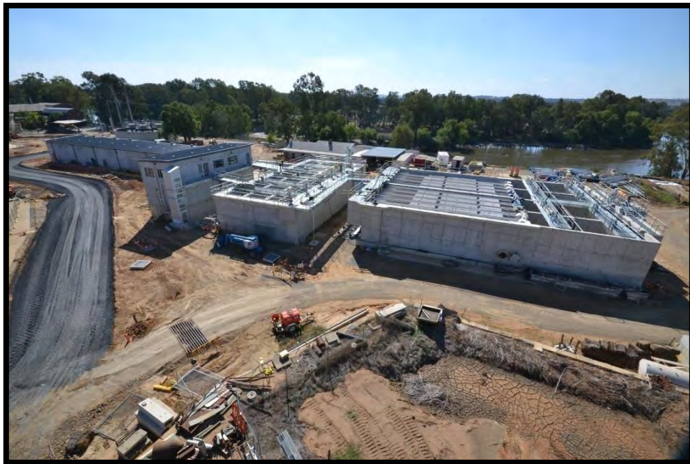
January 2017—Lamella Clarifier, Filter Block and Chemical Building with construction of stage 1 Roadwork
