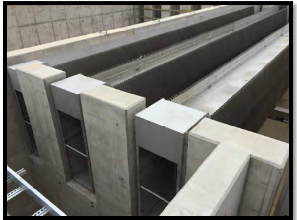
December 2016- Lamella clarifier trough installation
