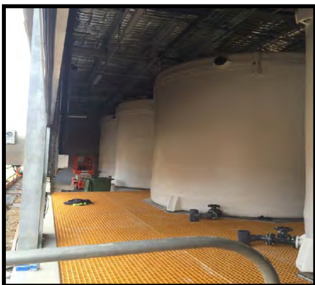
November 2016—Chemical Storage area grating installation
