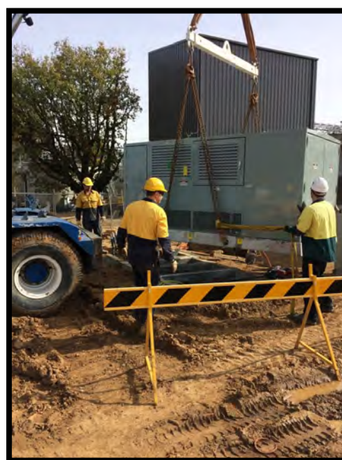
August 2016—Clearwater switchboard being placed into position
