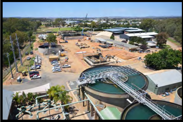
View of the lamella clarifier with the formwork removed from the flocculators. Filter cell walls are under construction.
