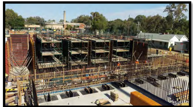
Backwash channel base being poured.
