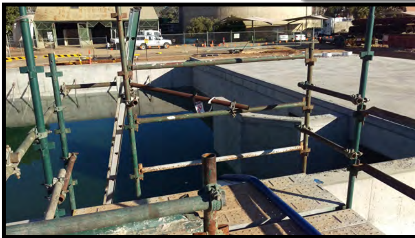
Clear Water Storage being filled to be hydro tested—the CWS tank is the last part of the water treatment process before the water is pumped into the distribution system
