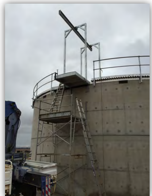
Installing ladder access
