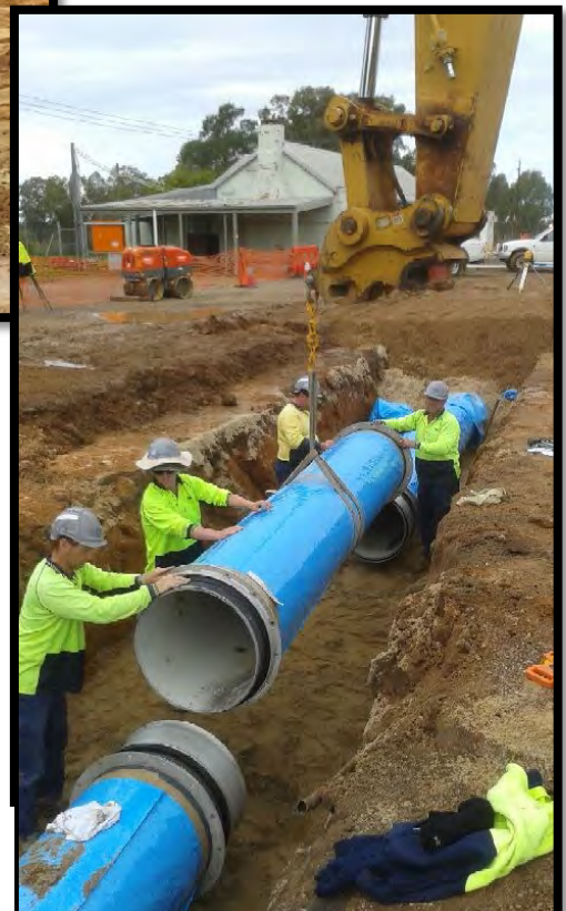
Riverina Water staff laying new pipework
