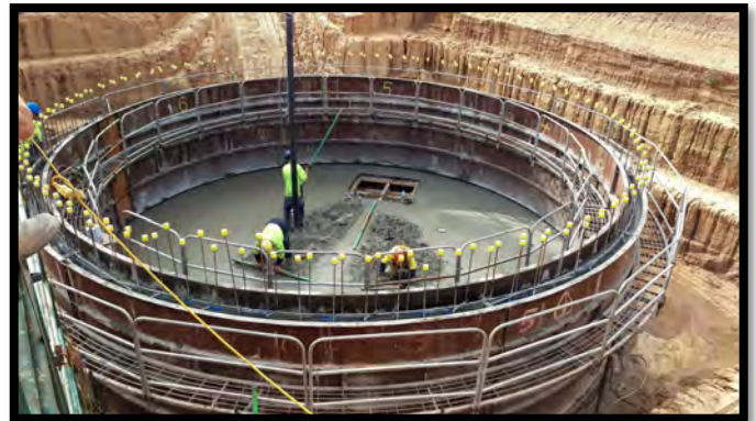
View of the construction of the Clearwater storage tank. The formwork for the northern walls is being installed.
