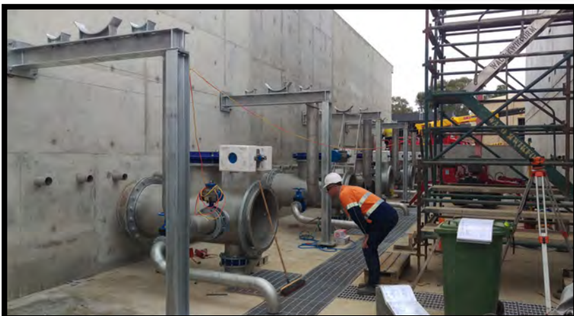
Mechanical Fitout of pipe gallery on the Filtered water tank—the tank collects water from filters before being transferred to the CWS tank.
