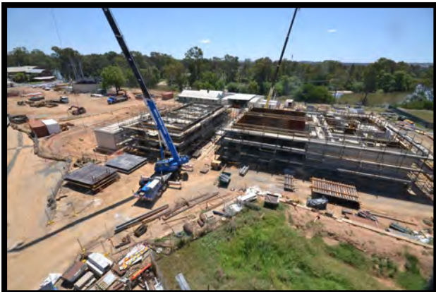
View of the filter cell formwork and scaffold being installed.
